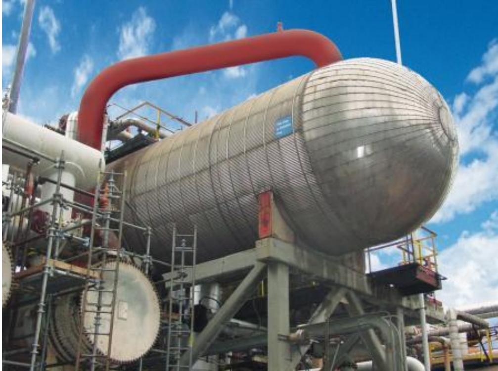
A column reboiler, or evaporator, is a heat exchanger that provides heat to the bottom of the distillation column. It boils the liquid at the bottom of the tower to produce vapor, which returns to the distillation column to drive the distillation separation process. A column reboiler may partially or completely evaporate the liquid collected at the bottom of the tower.
