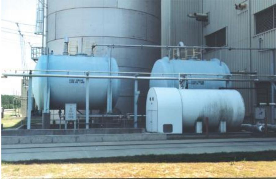
The generator and gas turbine have an integrated lubrication system to prevent damage caused by excessive friction. A part of lubricating oil is usually used in the hydraulic oil system. Lubricating oil is usually stored in integrated stainless steel and carbon steel tanks with level monitoring.
