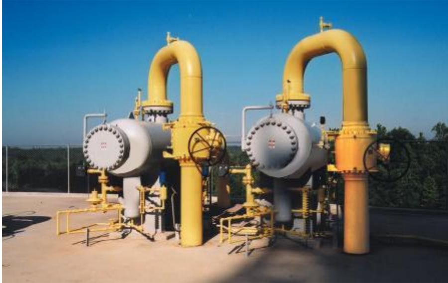
Natural gas separators can remove solid particles and liquids from a continuous gas stream, as well as dust, dirt, sand and pipeline scale, as well as water, natural gas liquids, and light hydrocarbons. In a typical system, the intake separator allows particles and liquid to settle and the gas to rise. The gas collected at the top of the separator is discharged through a gas compressor. The collected particles and liquid are then poured into a water tank.
