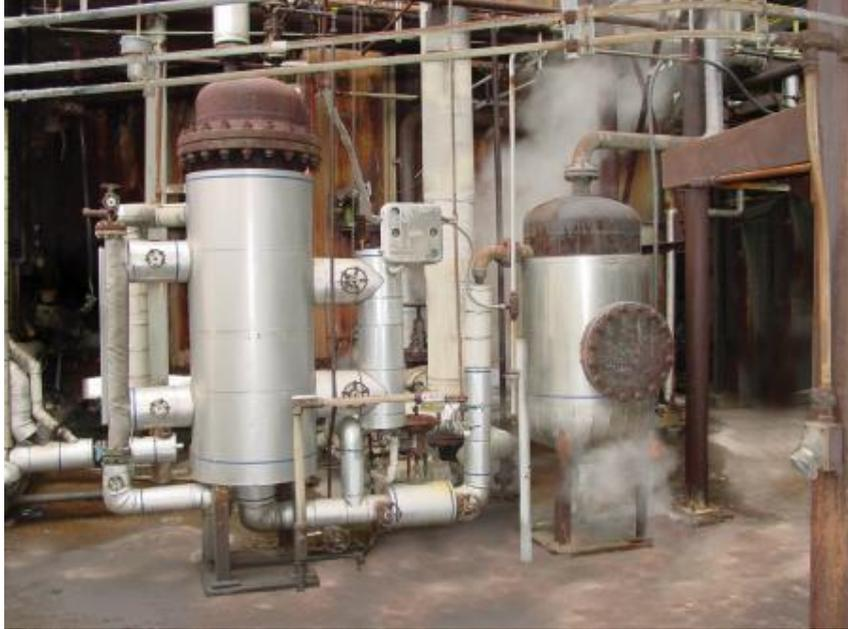
The heat exchanger extracts vapor from the upper part of the fractionator, cools it into liquid, and pumps it into the liquid reservoir (reflux tank). The liquid is then extracted from the bottom of the reservoir by a reflux pump, and a portion of the pump return (reflux) is reintroduced to the lower point in the tower. This reflux process improves the fractionator separation by ensuring sufficient liquid flow down to promote the vapor rise.
