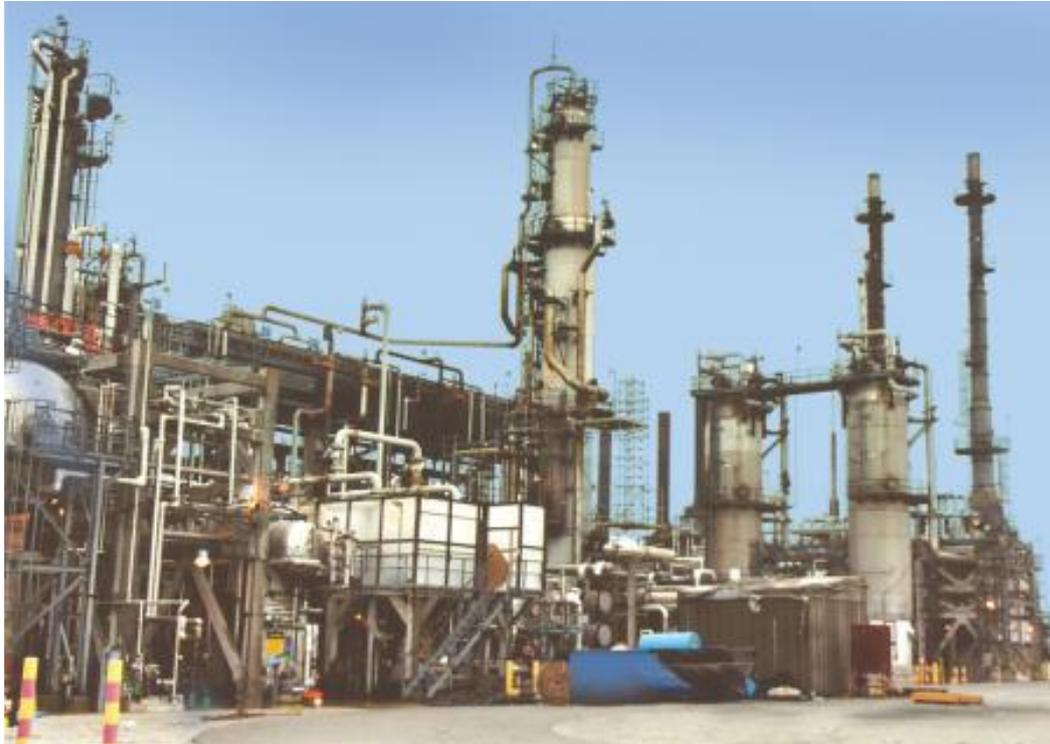
Catalytic hydrogenation is the treatment of liquid hydrocarbons in a hydrogen environment, through which 90% of impurities such as sulfur, nitrogen, oxygen and metal can be removed from the feed. The hydrotreating can also be used for the hydrodesorption of aromatic hydrocarbons (HDAr), hydrocracking of heavy diesel oil (HDHDC), dewaxing, and the performance improvement of cracking steam and diesel oil.
